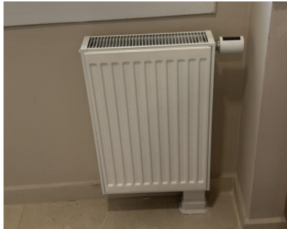
Figure 18. Smart thermostatic valve installation in Bayrampaşa
