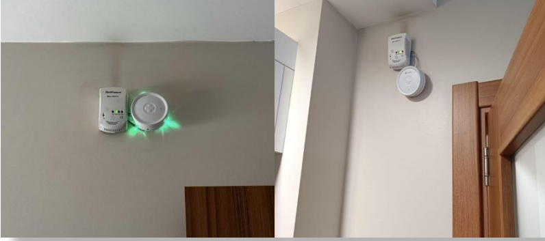
Figure 19. IAQ sensors & HVAC controllers in Bayrampaşa
